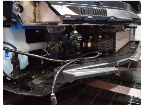
39. Adjust the pipe for best fitment then secure all remaining clamps.
